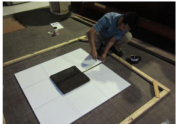
**Figure 8.** Attaching Pakis Blocks to Styrofoam
