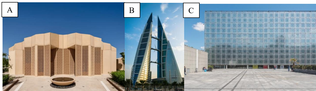
Fig. 2. Contemporary high-tech architecture incorporating elements of vernacular practices. A: Estidama Mosque, Abu Dhabi; B: Bahrain World Trade Center (BWTC), Bahrain; C: Arab World Institute Museum, Paris. Source: [(Parametric Architecture 2025)]
