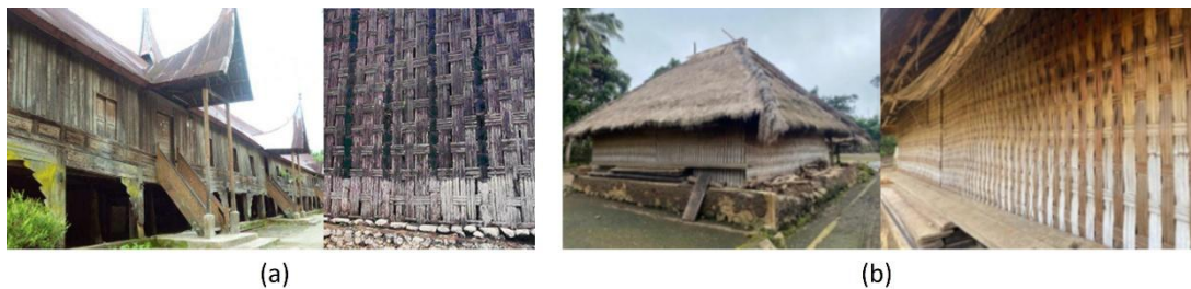
Fig. 3. Vernacular house, bamboo woven and wooden wall (a) Gadang house (b) Bale Mangina (Source: Anthony S. Rares, 2025; Saptaningtyas et al., 2025)
