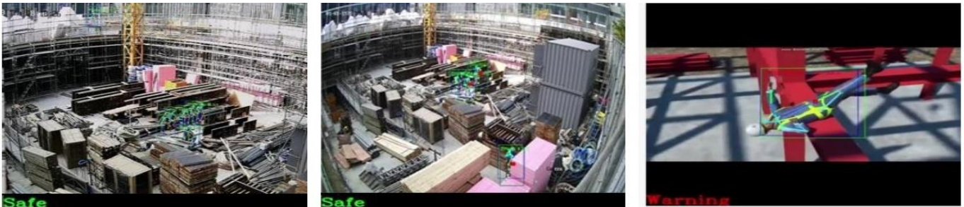
Fig. 11. The AI Model for Detecting Falls Among Workers was Demonstrated at the Construction Site Source: J. Lee and Lee, 2023
