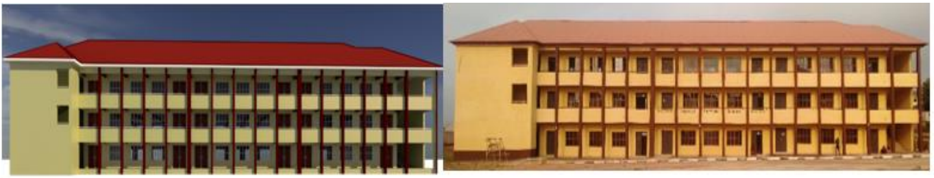
Fig. 3. Approach View of the Classroom Block- Model (Left), Field Snapshot (Right)
