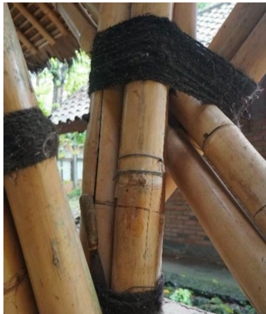
Fig. 2. Bamboo rope joinery (Dewagana & Arif, 2022)
