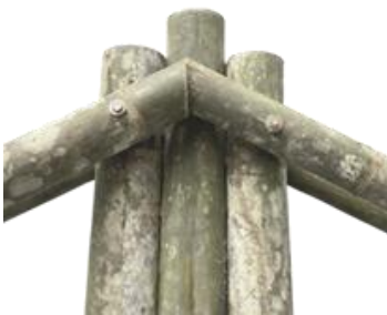
Fig. 15. D point joinery detail
