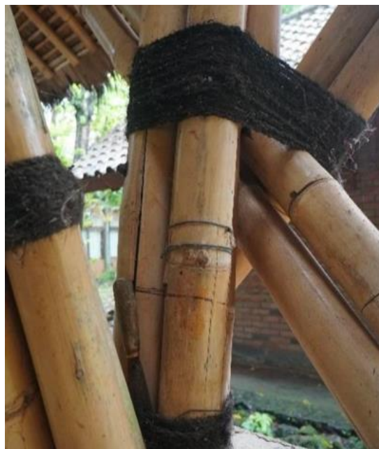
Fig. 2. Bamboo rope joinery (Dewagana & Arif, 2022)
