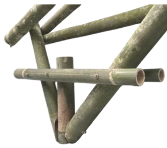
Fig. 19. A and G point joinery detail
