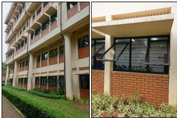
Fig. 4. S Building South Façade & Windows
