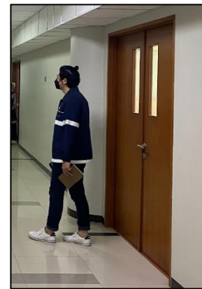
Fig. 5. Two leaves double-acting door
