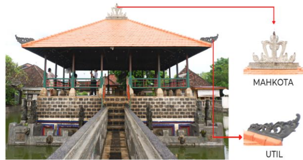
Fig. 11. The use of roof mahkota and util on the roof of Bale Kambang as a characteristic of Balinese architecture.
