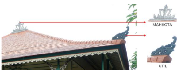
Fig. 7. Mahkota and Util ornament on the roof of Gedong Maskerdam
