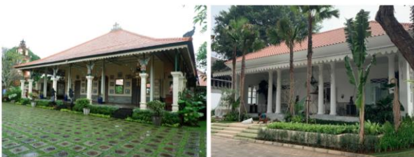
Fig. 3. Gedong Maskerdam (left) and an example of a colonial style building (right) (Source: Kompas.com)
