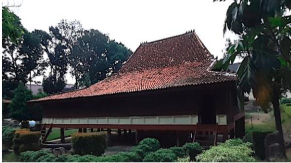
Fig. 2. Front View of Limas House
