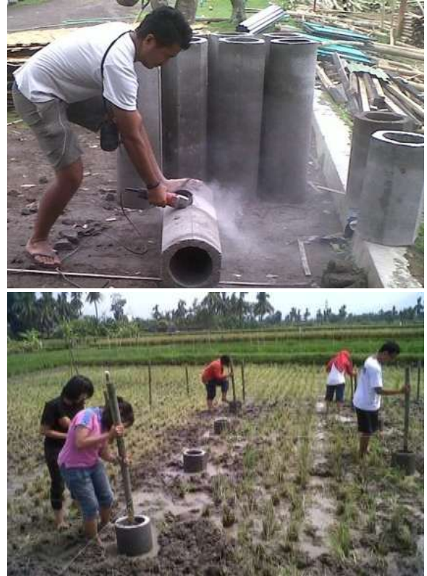
Fig. 2. Hollow Pedestal Foundation Construction Process and Placement on the Site
