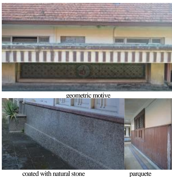
Fig. 5. Walls of M. Asngad's Family Residence (Source: Primary Survey, 2017)
