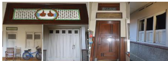
Fig. 7. Opening of M. Asngad's Family Residence (Source: Primary Survey, 2017)
