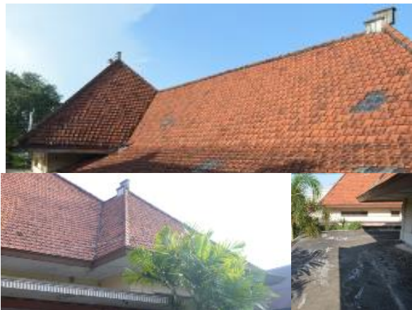
Fig. 4. Roof of M. Asngad's Family Residence (Source: Primary Survey, 2017)
