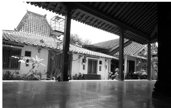
Fig. 4. Traditional House ( dalem/omah ) view from Pendopo Building in Kotagede
