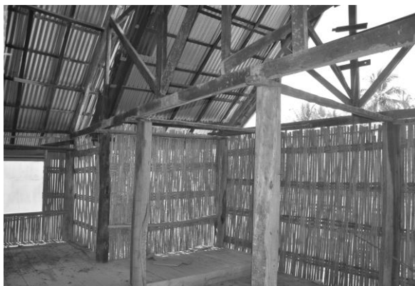
Figure 9. Wall structure weaved from bamboo
