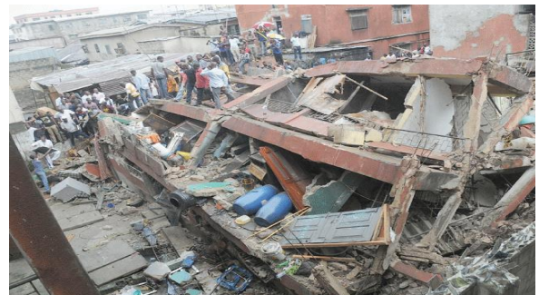
Figure 4. Building collapse in Lagos. (Source: http://daily-post.com.ng/wp-content/uploads/2013/07/Lagos_collapsed_building.if )
