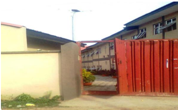
Plate 2. A Students' Hostel with inadequate setbacks, perimeter fence and landscaped with a mix of hard and soft landscape elements.
