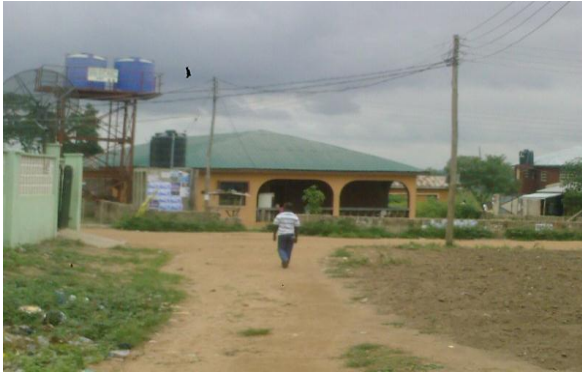
Plate 1. A Students' Hostel with inadequate front setback, without perimeter fence and poorly landscaped open spaces.
