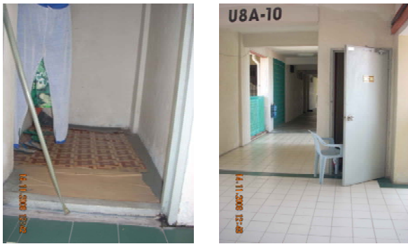
Figure 2: Internal view of experimental room and entry of the room
