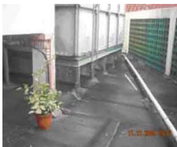
Bare roof top before Greenery
