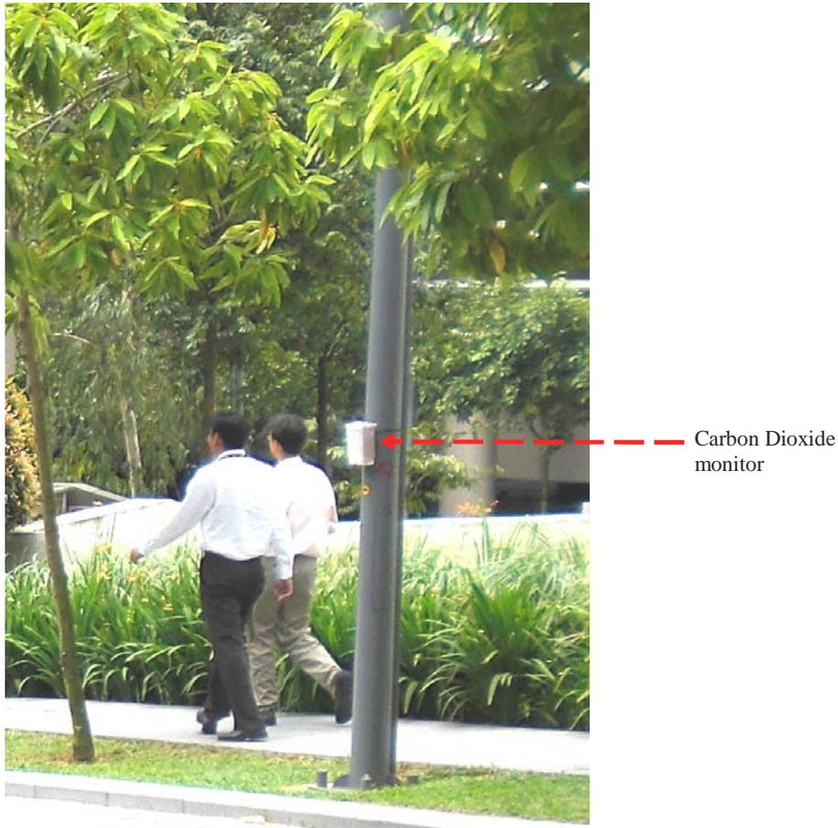
**Figure 2.** CO<sub>2</sub> sensor installations
