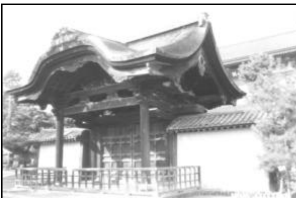
Figure 13. The Chokushimon (Imperial Messenger Gate). It was constructed in 1590, it is an example of the curved-gable style of the Momoyama period.
