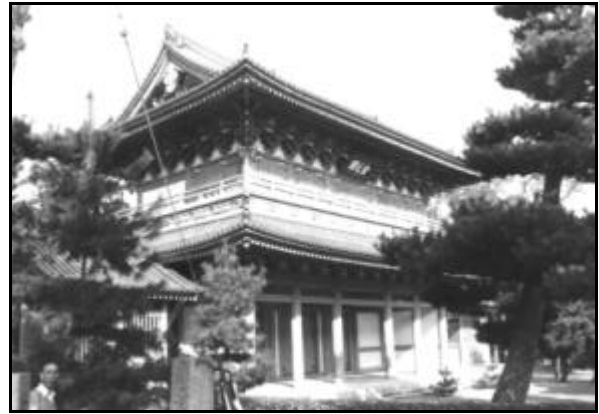
Figure 14. The sanmon of Daitoku-ji Monastery, The Upper Story was added by the tea Master Sen no Rikyū in 1589.
