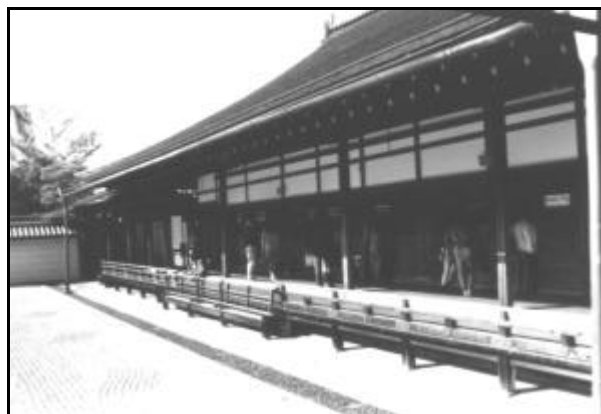
Figure 3. The Hōjō of Nanzen-ji monastery, it was erected in the Tenshō era (1573-1591).
