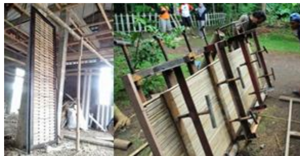
Fig. 7. Level of prefabrication in Kampung Naga's house
