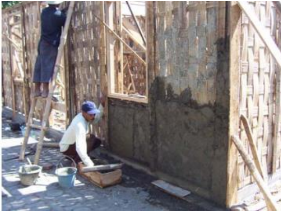
Figure 7. The making of plastered bamboo wall
