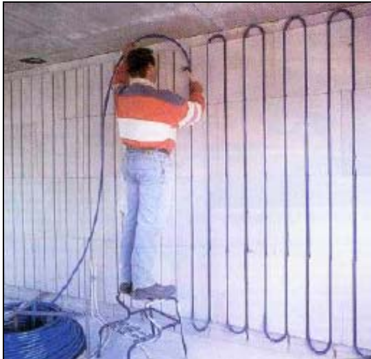
Figure 2. Wall heating low quality energy that stored in the Ground. (Schmidt, 2001)
