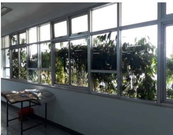
Fig.4. Window opening, West orientation on 15 May 2019, 15.00
