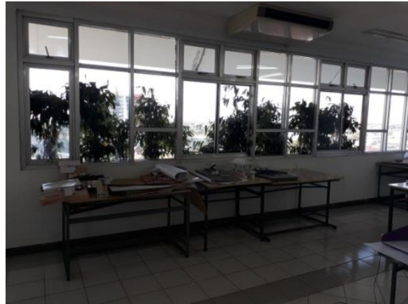
Fig. 5. Window opening, South orientation on 15 May 2019, 15.00
