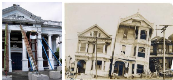
Fig. 1. Structures with heavy materials will always vulnerable to earthquakes New Zealand 2011 and the surviving wooden structure did not collapse instantly in the event of the 1906 San Francisco earthquake (photo: Martin Luff and US National Archives).
