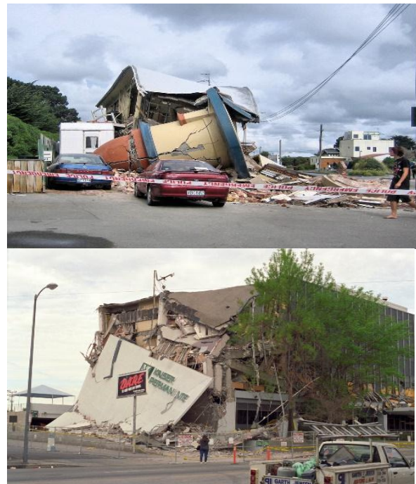
Fig. 6. The failure of heavy elements on the upper floors such as tower roof (left) and wall element (right) in Christchurch 2011 earthquake (photo: Martin Luff)
