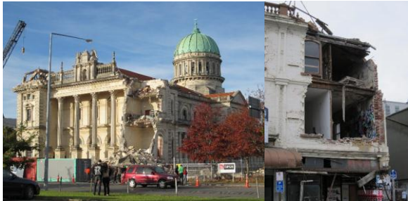
Fig. 7. Damage in the outer elements are generally occurs in the corner of the building (photo: Martin Luff)
