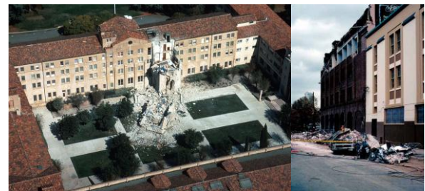
Fig. 3. The adjacent buildings will destroy the weaker one (photo: Wilshire and Meyer USGS)
