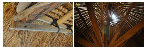
Fig. 8. Some modern modification; (a) Bamboo nailed at rafter (b) Square wooden beams encircling central pole of Mbaru Niang
