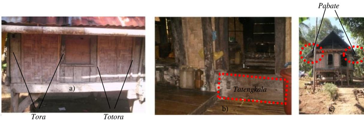
**Fig. 6.** *Tora, totora, tatengkala, and form of pabate made tiangle* (Source: Umar, 2012).
