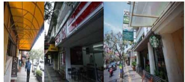
Fig. 9. Adaptation Process in Old Building for Increase the Comfort Zone
