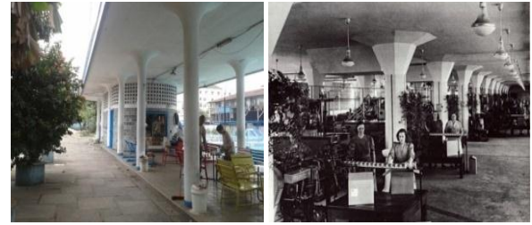
Fig. 13. Concrete Mushroom Column on Paradiso Swimming Pool and Van Nelle factory (Source: Personal and Facilitaire-info)
