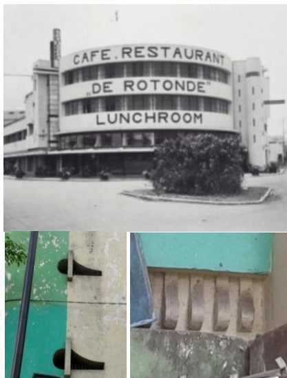
Fig. 7. The Form of the Building and the Expressive Ventilation on Facade and there was Ornament on Façade (Source: Tropenmuseum)
