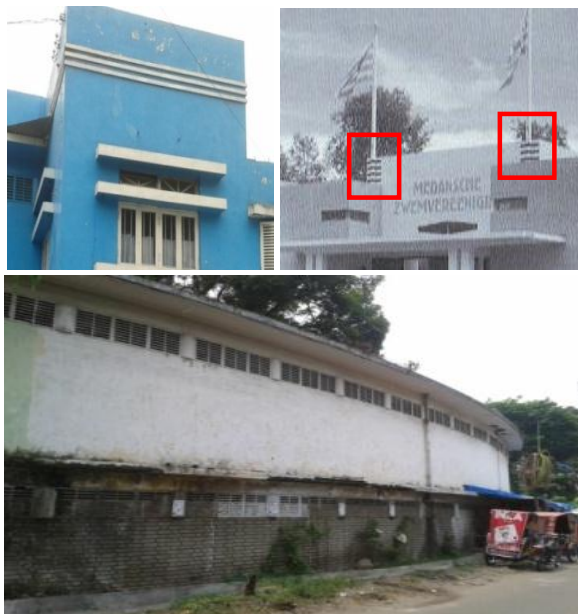
Fig. 12. Ornament on front Facade and Brick was not plastered on side wall (Source: Samedan)
