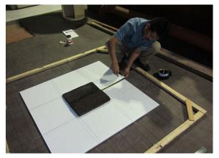
Figure 8. Attaching Pakis Blocks to Styrofoam
