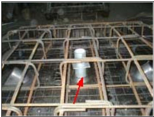
Figure 10. Cast-in socket
