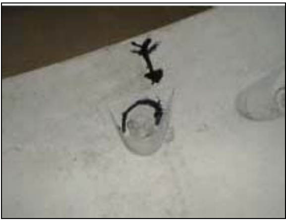
Figure 12. Displacement of plastic sheath
