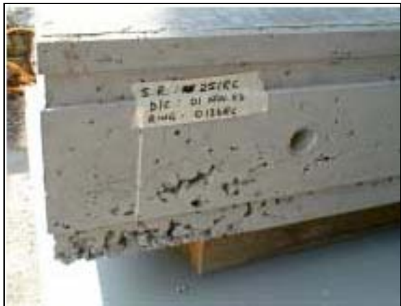
Figure 11. Honeycombing
