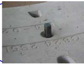
Figure 15. Metal bolt in cast-in socket
