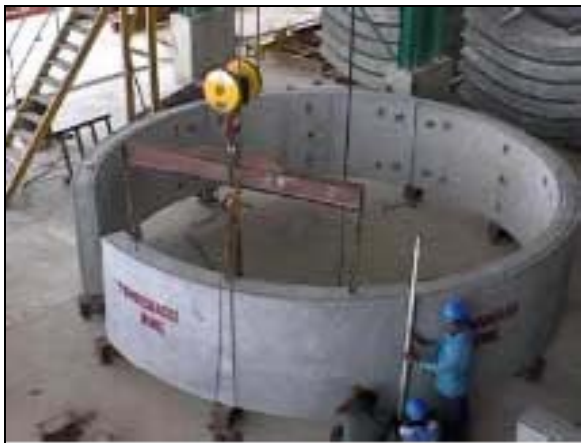
Figure 16. Trial ring installation
